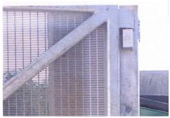
Hinges should be located on the outside of the frame to allow maximum opening of the gates/doors. Hinges must be heavy-duty to withstand regular use. Recology will not be liable for hinge failure due to normal wear and tear.
