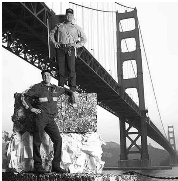
Recycle Central, a new MRF in San Francisco, made its debut earlier this month. The facility, which overlooks the Golden Gate bridge, processes up to 2,100 tons of recyclables per day.
